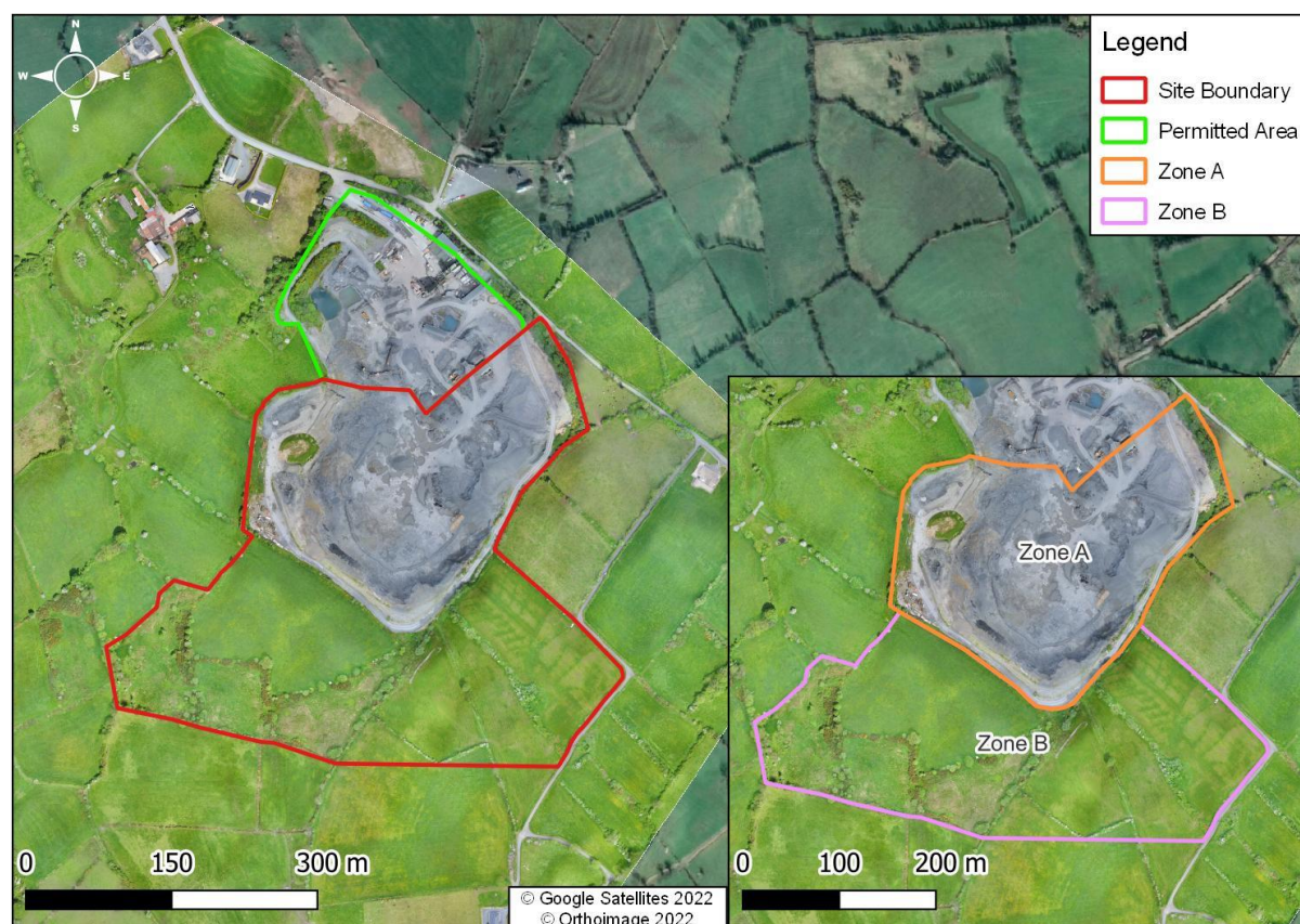
Figure 3-2: Overview of Site
